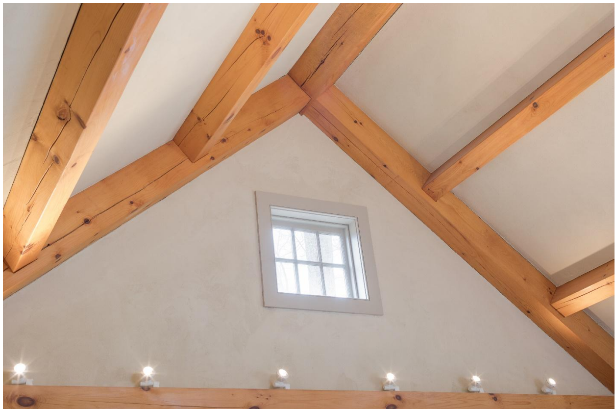
Light fixtures mounted on top of timbers bounce light off a plaster ceiling
