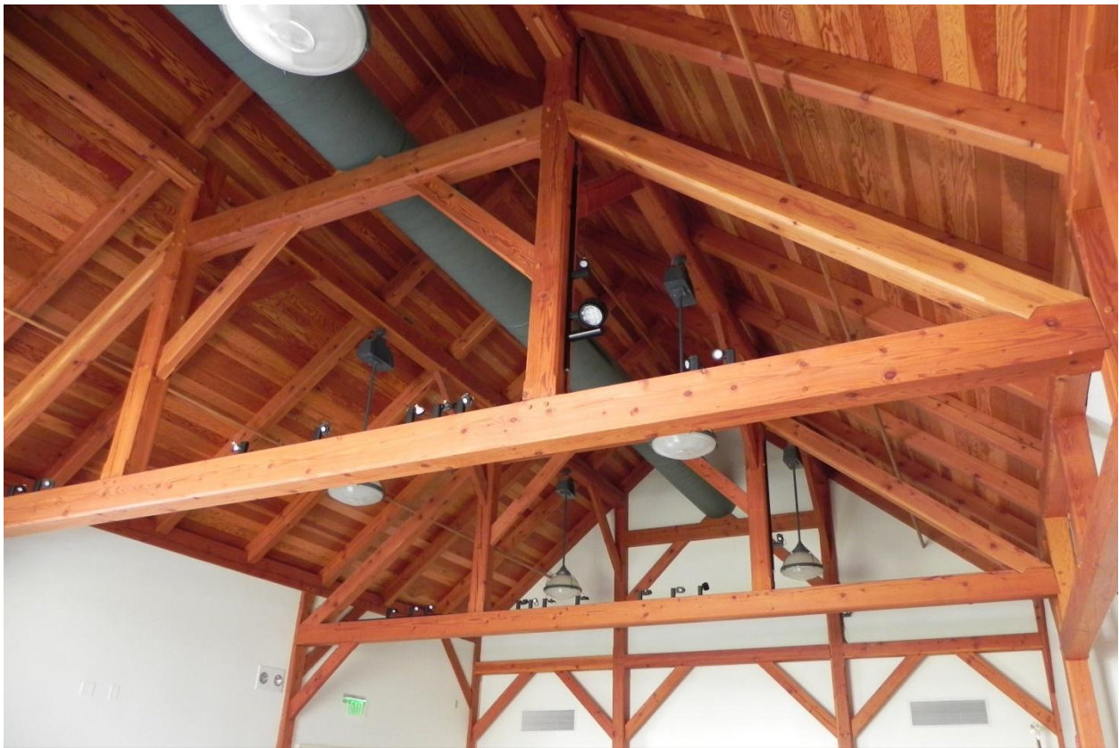
Douglas Fir queen post trusses
