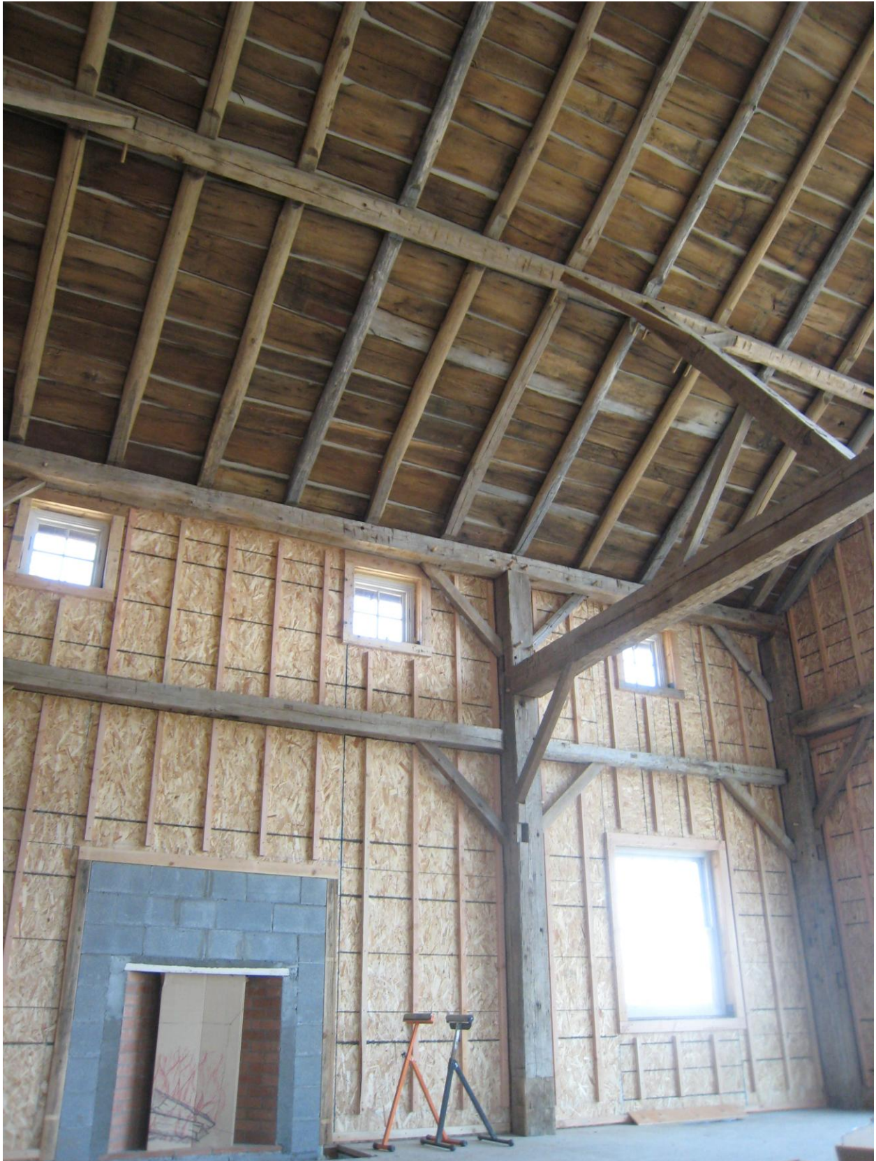
SIP panels enclose and help support a restored timber barn frame
