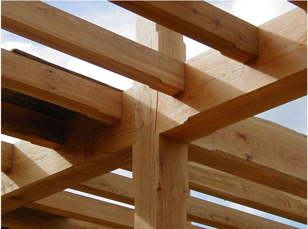
Chamfered timbers with “ski tip” stops on the joists and “lamb’s tongue” stops on the posts and beams
