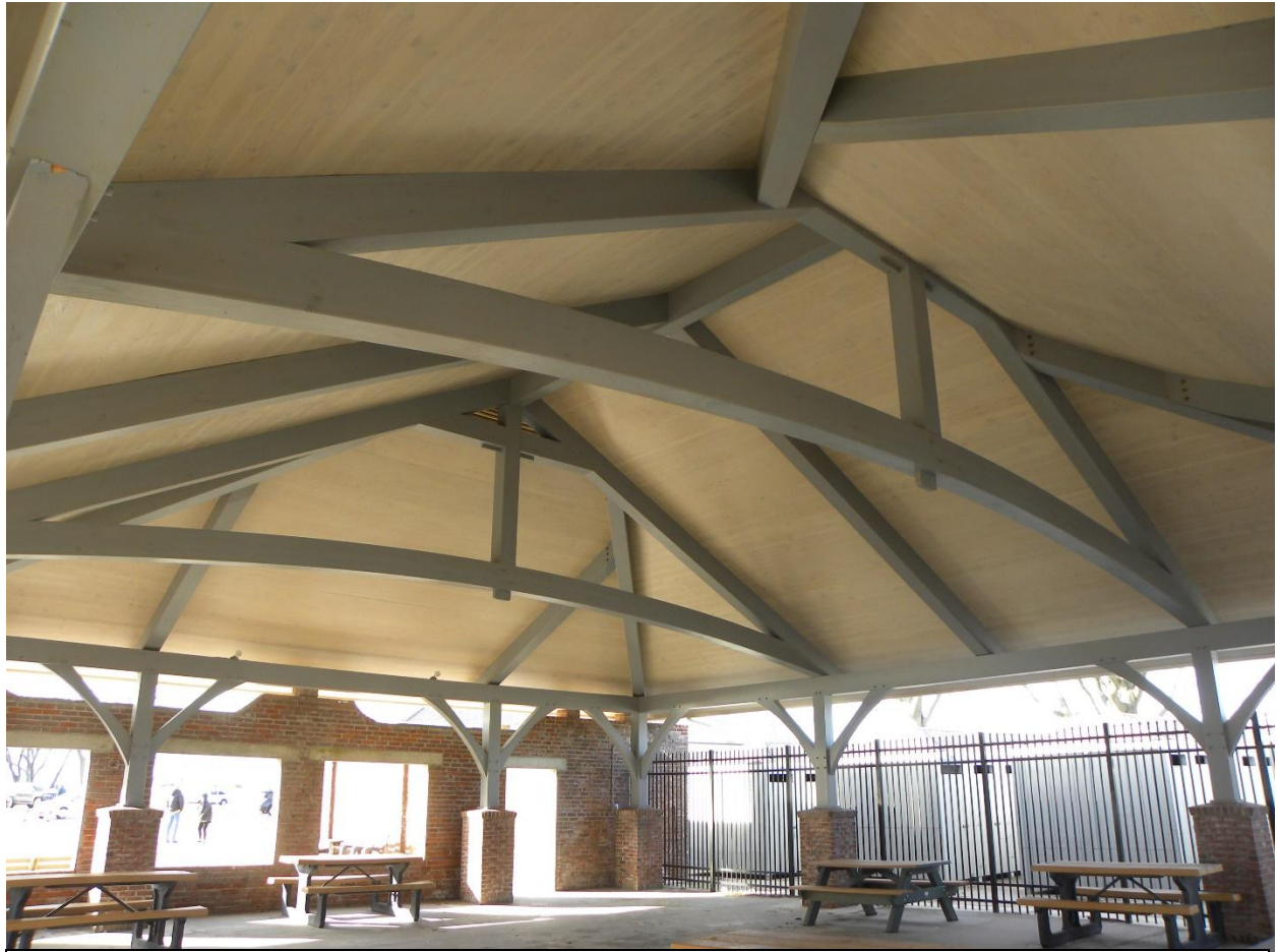
The Compo Beach Pavilion in Westport, CT features CLT panels over glulam trusses with traditional joinery
