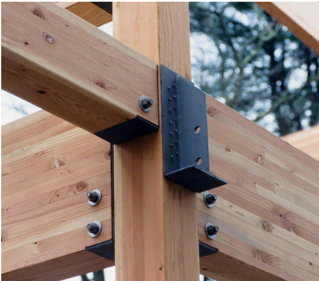
This stiffened seat connection is secured to the timber column with timber rivets
