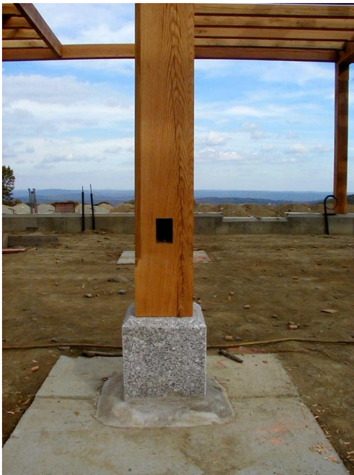
Granite plinth keeps the timber post base high and dry
