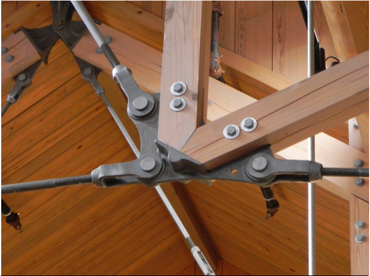
Custom cast steel connection hardware can produce elegant timber connections
