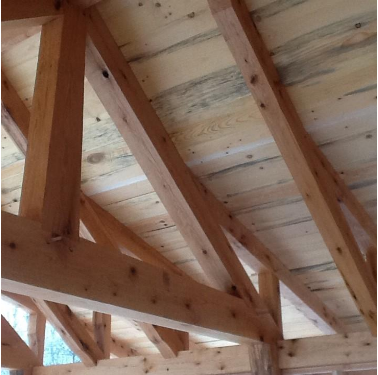
Red Oak king post truss with Denim Pine ceiling
