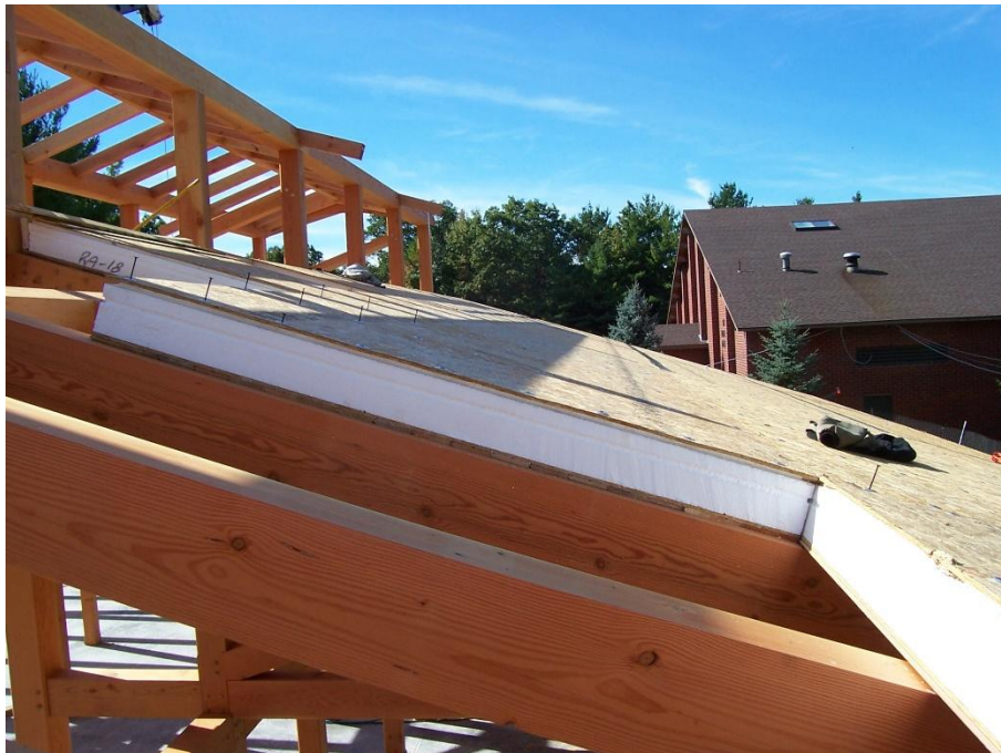
SIPs with XPS core (pink) and EPS core (white)
