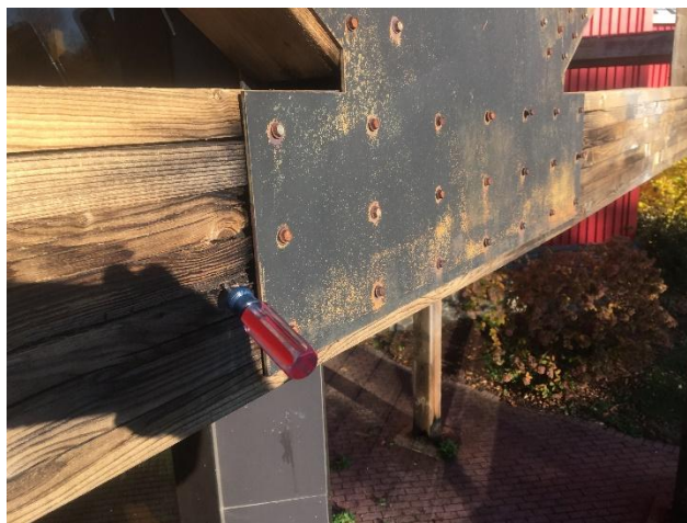
Fungal decay behind an exposed gusset plate
