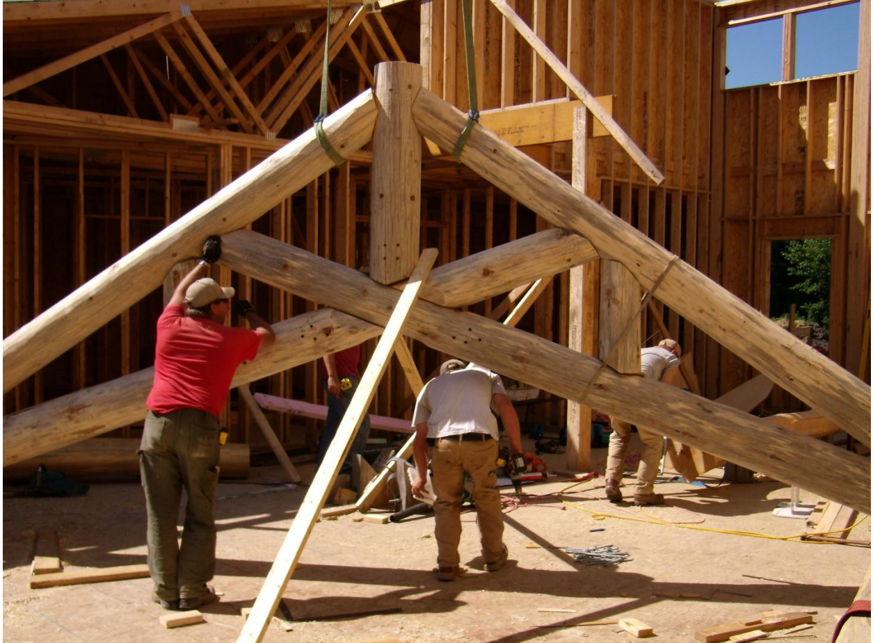
Log scissor truss
