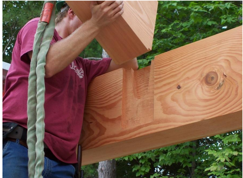
Rounded dovetail joints are easy with CNC fabrication
