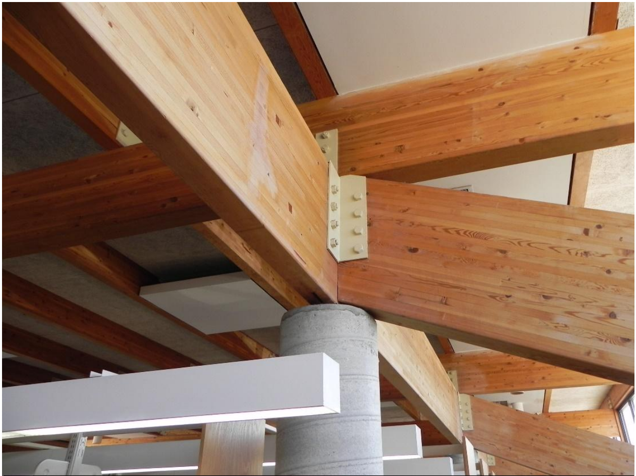
Traditional style engineered glulam connections
