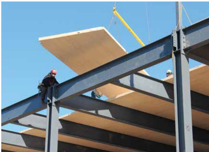
Figure 5. Cross-laminated Timber (CLT) panels being erected over a structural steel frame.
