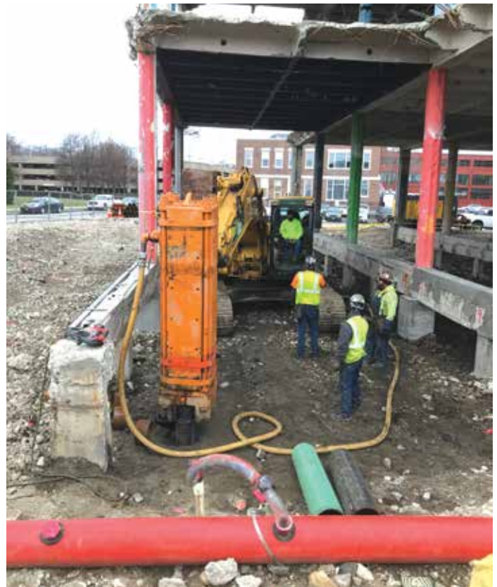
Figure 3. Custom pile driving rig.
