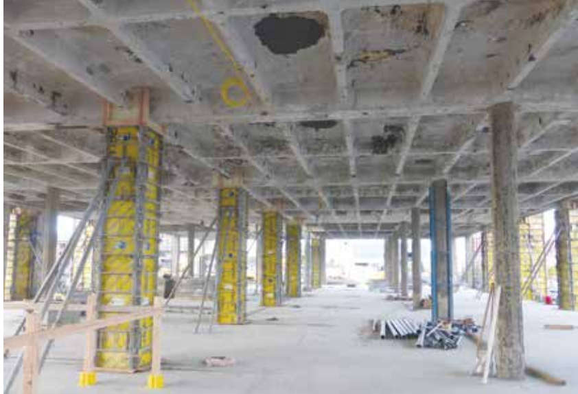
Figure 4. Concrete columns were reinforced and jacketed to increase capacity.
