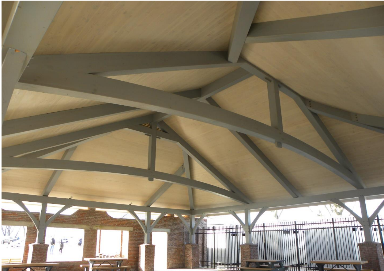
Glulam trusses with curved bottom chords
