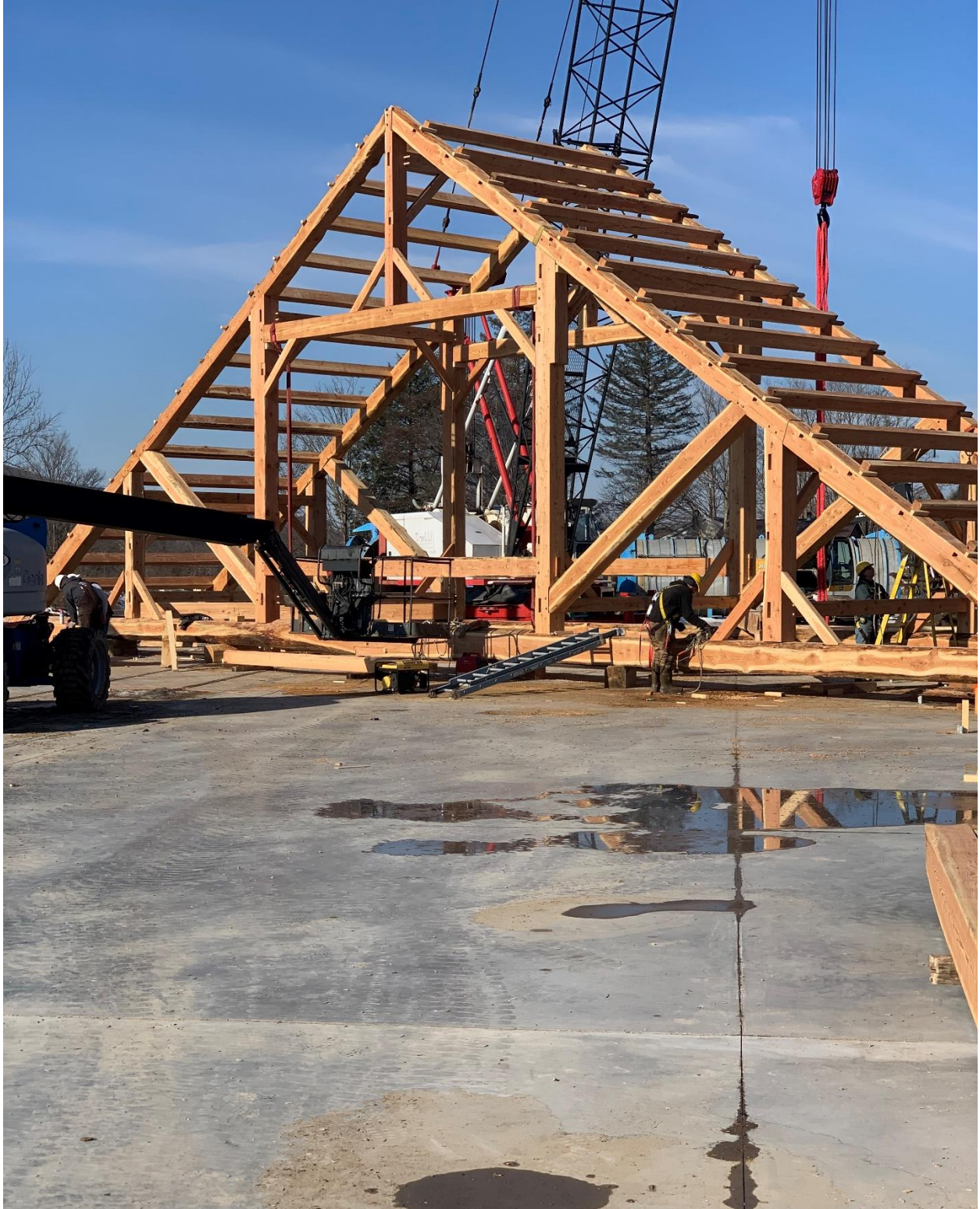
80-foot span queen-post trusses
