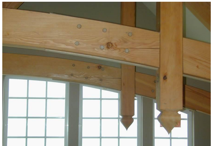
Seasoning checks indicate the grain orientation.
