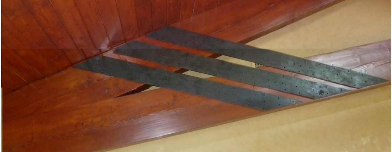
Straps on repaired scissor truss – basically, the aspect ratio of this plate and its connectors makes it behave more like a single axial strap (or, even, akin to a fully-threaded screw)
