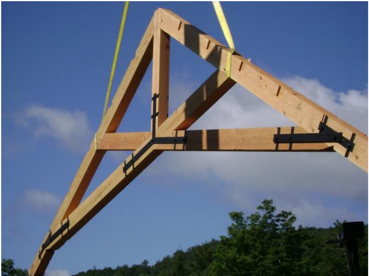
Pinned straps on scissor truss
