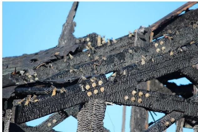
Protecting timber connections with gypsum board is seldom an acceptable approach for an architecturally exposed timber structure.
