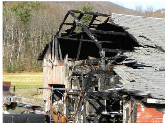
When timber structures do eventually fail during a fire, they often do not fail suddenly. They sometimes give warning signs such as making loud cracking and hissing noises when a collapse is imminent. Timber connections with unprotected steel hardware, however, can fail suddenly without warning. Consequently, careful detailing of timber connections is crucial.
