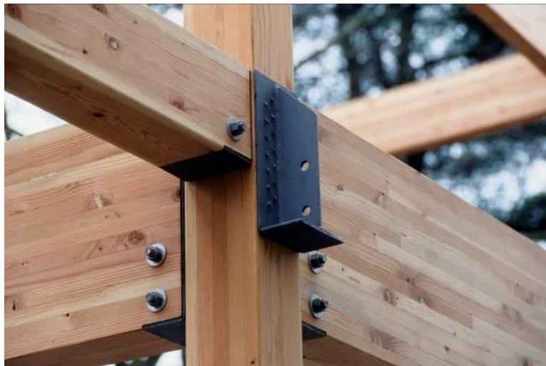
Figure 3 Connection hardware is shop fastened with timber rivets and field bolted. The beam reaction is resisted in bearing on the seat and the bolts are not taking load.
