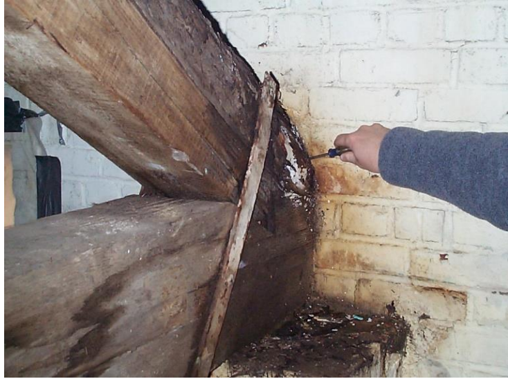
Figure 13 An awl is used to probe for rot.
