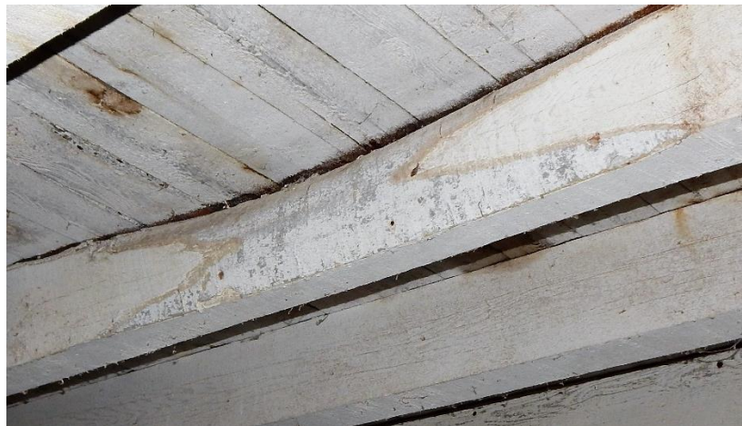
Figure 30 Excessive wane that exceeds grading rule limits
