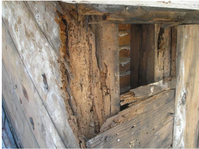
Figure 5 Termite damaged timber
