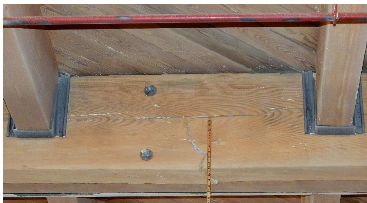
Figure 29 Fracture terminating at a check
