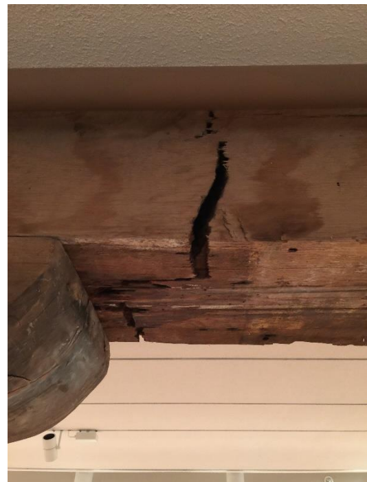
Figure 8 Fractured timber due to overloading
