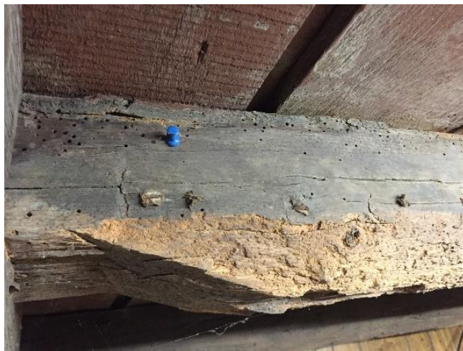
Figure 6 Powder post beetle damage
