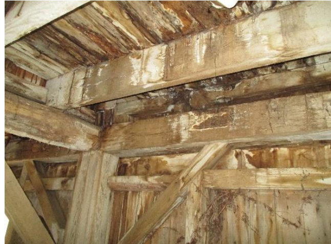
Figure 3 Discoloration can be a sign of rot
