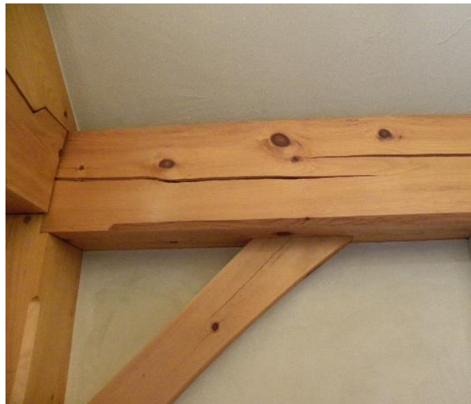
Figure 18 Seasoning checks are not material defects
