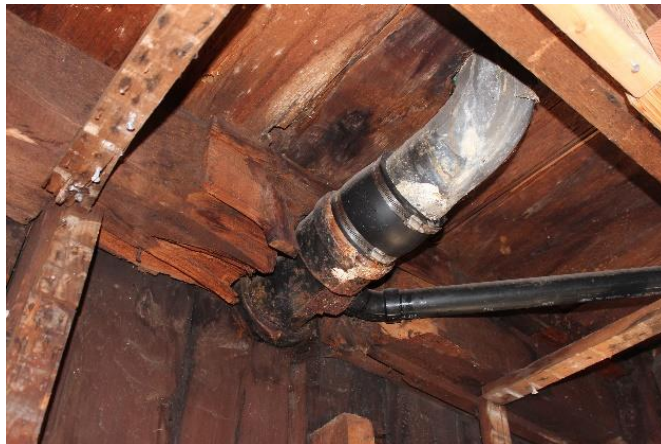
Figure 7 A timber that has been compromised
