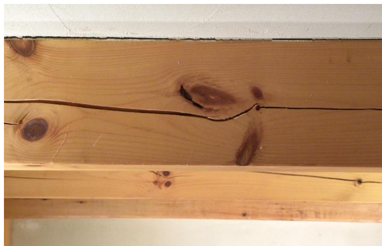
Figure 28 Grain deviation at knots
