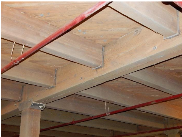
Figure 25 Blast cleaning of timbers makes grading more reliable
