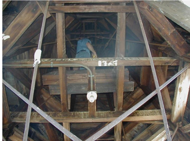
Figure 24 Evaluation and grading of timbers in a church steeple
