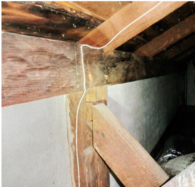
Figure 17 Shear failure in the tenon (relish failure) of a rising brace
