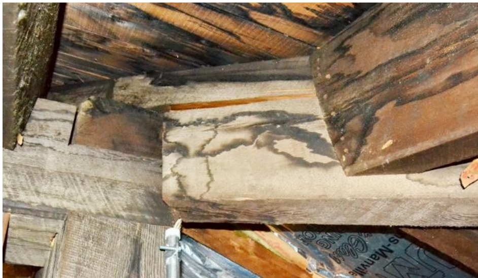
Figure 10 Split in a notched timber
