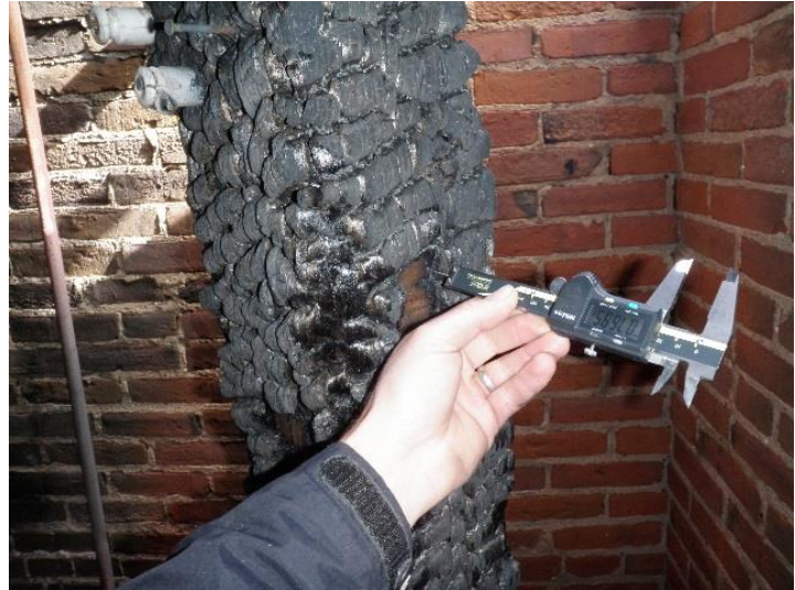
Figure 11 Fire damaged timber
