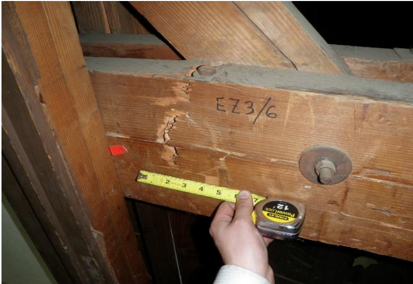
Figure 9 Tension fracture in bottom chord of a bowstring truss
