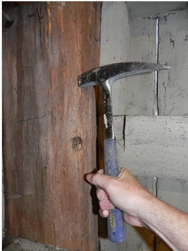
Figure 14 A rock pick can be used for sounding
