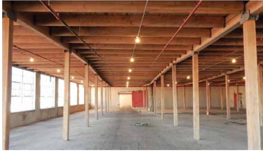
Older timber structures are easily adapted to a variety of uses.
