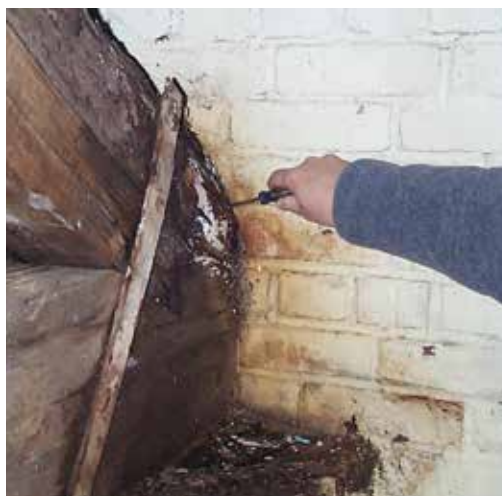
An awl is an effective tool for evaluating surface deterioration.
