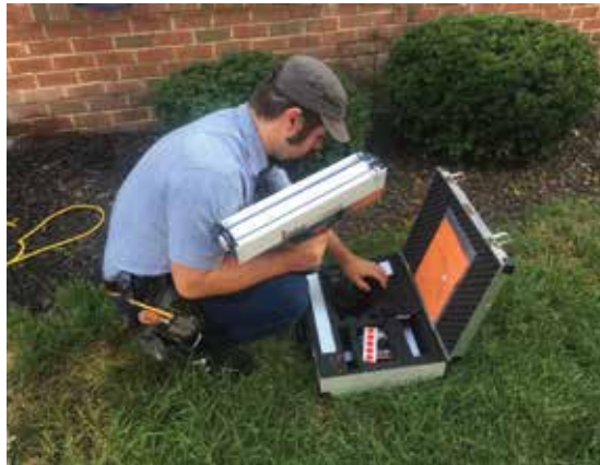
A resistance drill can identify hidden deterioration within a timber.
