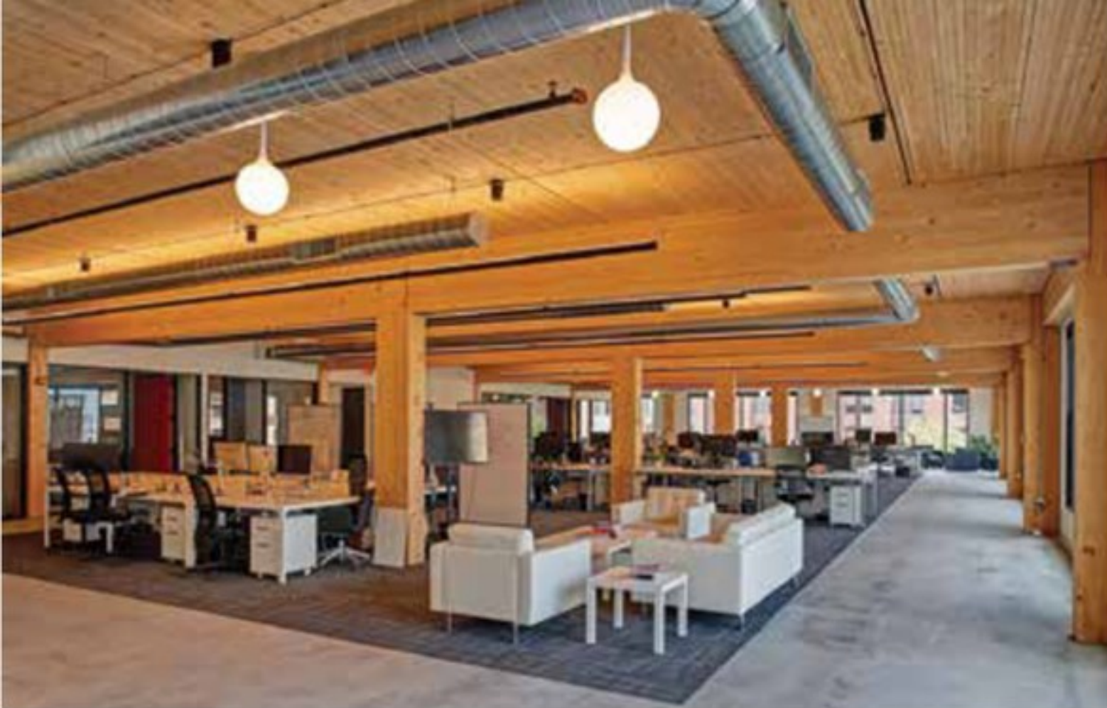
T3 Office Building's Nail Laminated Timber panels on glulam framing. Courtesy of Bergerson Photography.
