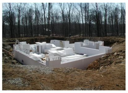
Top: Lite Deck ICFs installed for concrete beams and floor slab. Bottom: Foundation walls installed with ICFs, concrete not yet placed.
