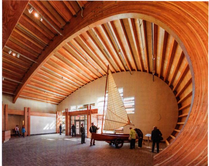
to create a seamless-looking roof. Floyd is particularly pleased by the lack of exposed steel inside the building—steel knife plates, used to connect the glulam structural members, are cut into the members, giving the project "a much more elegant effect," he says.
