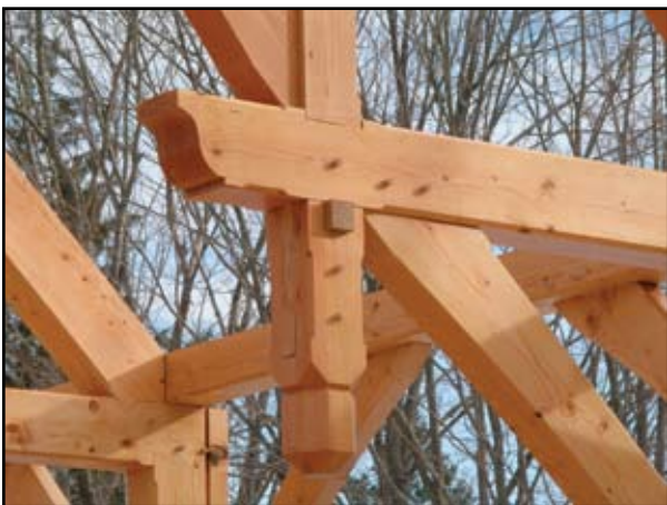
Hammerbeam joint. Courtesy of Kevin H. Chamberlain.
