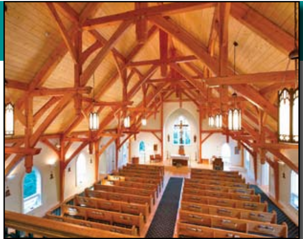
Church interior with exposed timber frame. Courtesy of Olson Photographic, LLC.
