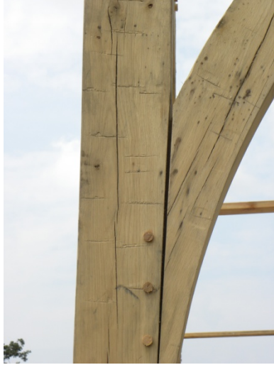
Figure 3 - Knee Brace Joint
