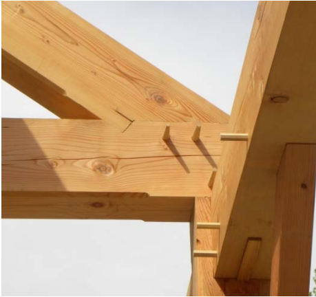
Figure 1 - Truss Heel Joint
