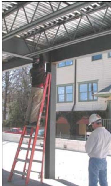
need to be solvent cleaned to remove oil left on the surface after galvanizing operations.
