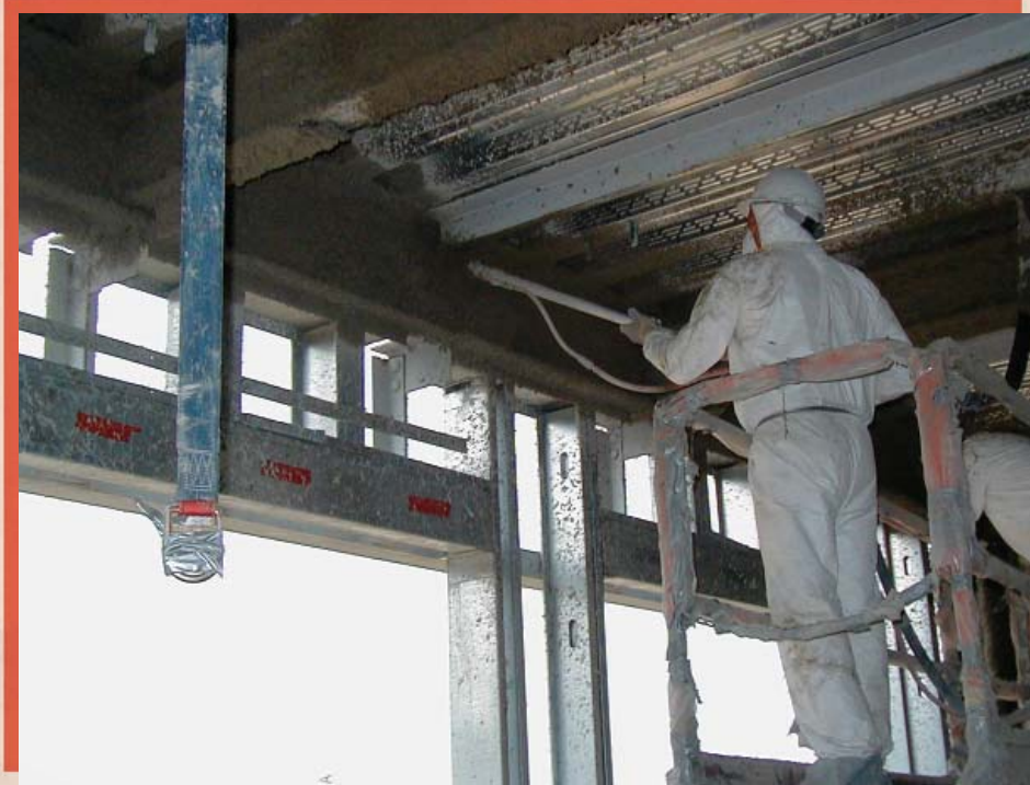
Application of fireproofing
