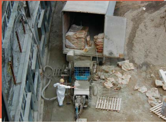
Fireproofing mixer and pump
