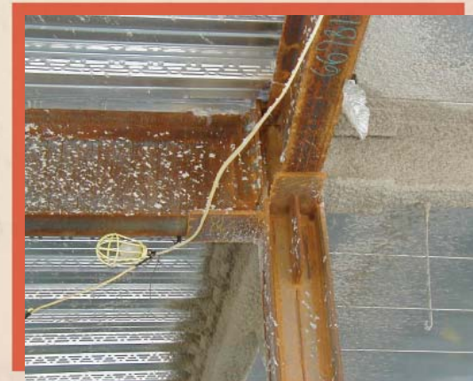
Fireproofing should be applied to bare unpainted steel
