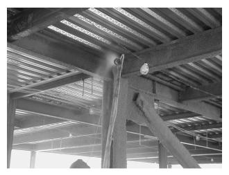
deck are completely filled over beams. During cold weather, precautions need to be taken to allow proper curing conditions and to prevent the material from freezing. Adequate ventilation is required during curing to allow moisture to be removed from the air and to prevent mold growth in the fireproofing.
